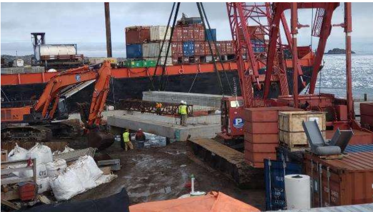
Pier Construction in February 2022. Image Credit: Marissa Goerke
