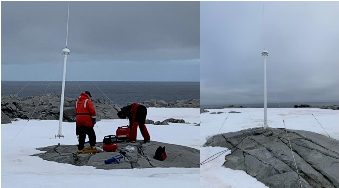
Fig. 3 – The Kohut team (along with ASC assistance) prepares to move the Wauwermans Island HFR antenna to newly exposed bare rock (left panel), and the mounted antenna two days later (right panel). Image Credit: Kohut group
