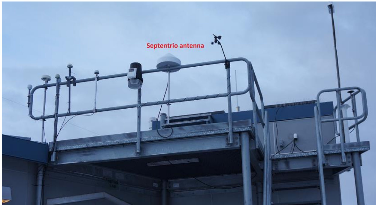
Figure 1. GPS antenna installation on the roof of the Terra Lab building.
